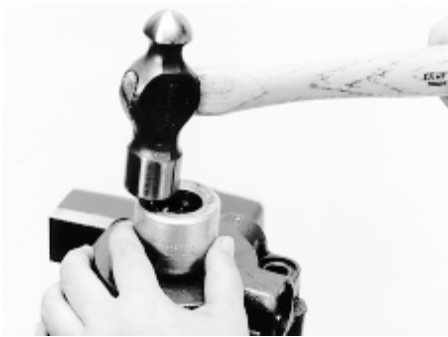
Install input shaft seal
