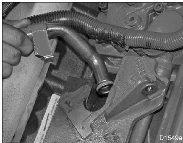
Figure 59 Removal of oil drain tube for VGT
