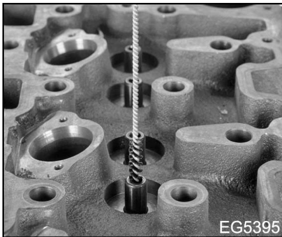
Figure 97 Clean valve guides
