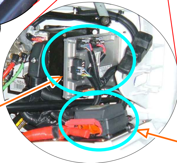
Power Distribution (Module 285 PDM)
